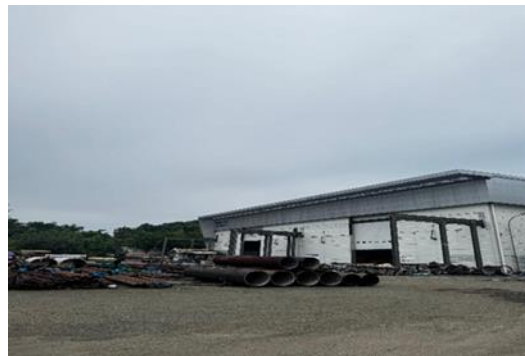
Gambar 3 Material Pipa Baja Di Area Depan Warehouse
